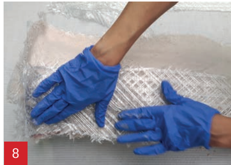
...and apply a 2nd layer of A1 Triaxial fibre on the still wet A1.
