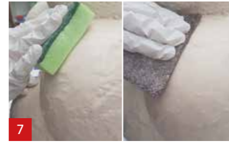
7 Or use (after ±20 minutes) a damp sponge or a waterproof sanding pad.
