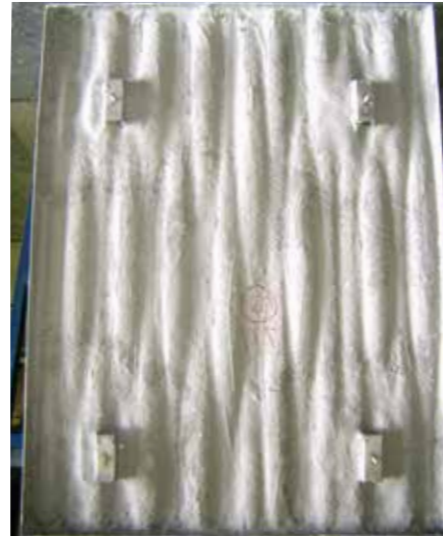
Panels Protea building - South Africa
