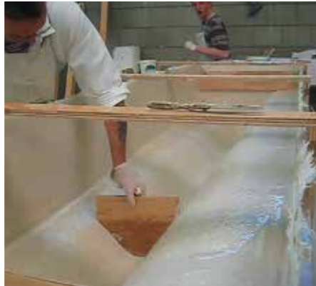
Construction inside panel Mahler - The Netherlands
