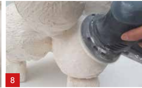
8 Or by using sanding paper manually or by machine.
