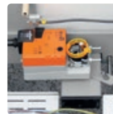
Automatic air supply and exhaust air flaps
