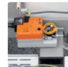
Automatic air supply and exhaust air flaps
