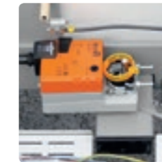
Automatic air supply and exhaust air flaps
